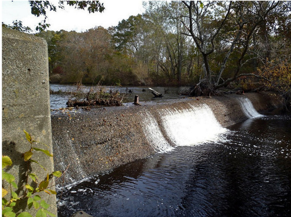
Concrete structure Removed 2015
