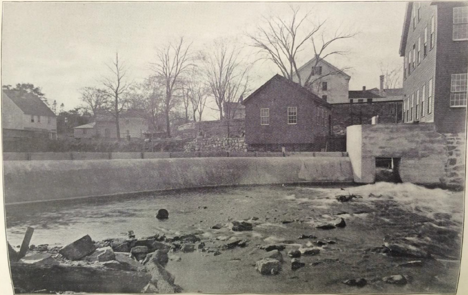
POTTER'S HILL DAM.—Dam and Waste Gate, looking up stream.
