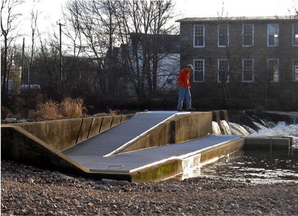
Existing Fish Ladder Possibility for removal
