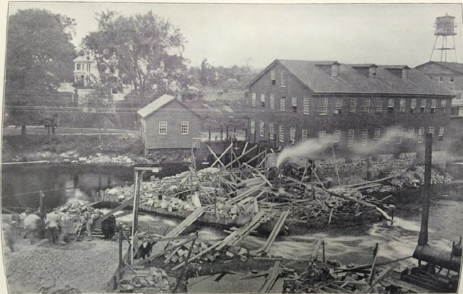
POTTER'S HILL DAM.—During construction of Waste Gate Abutment.
