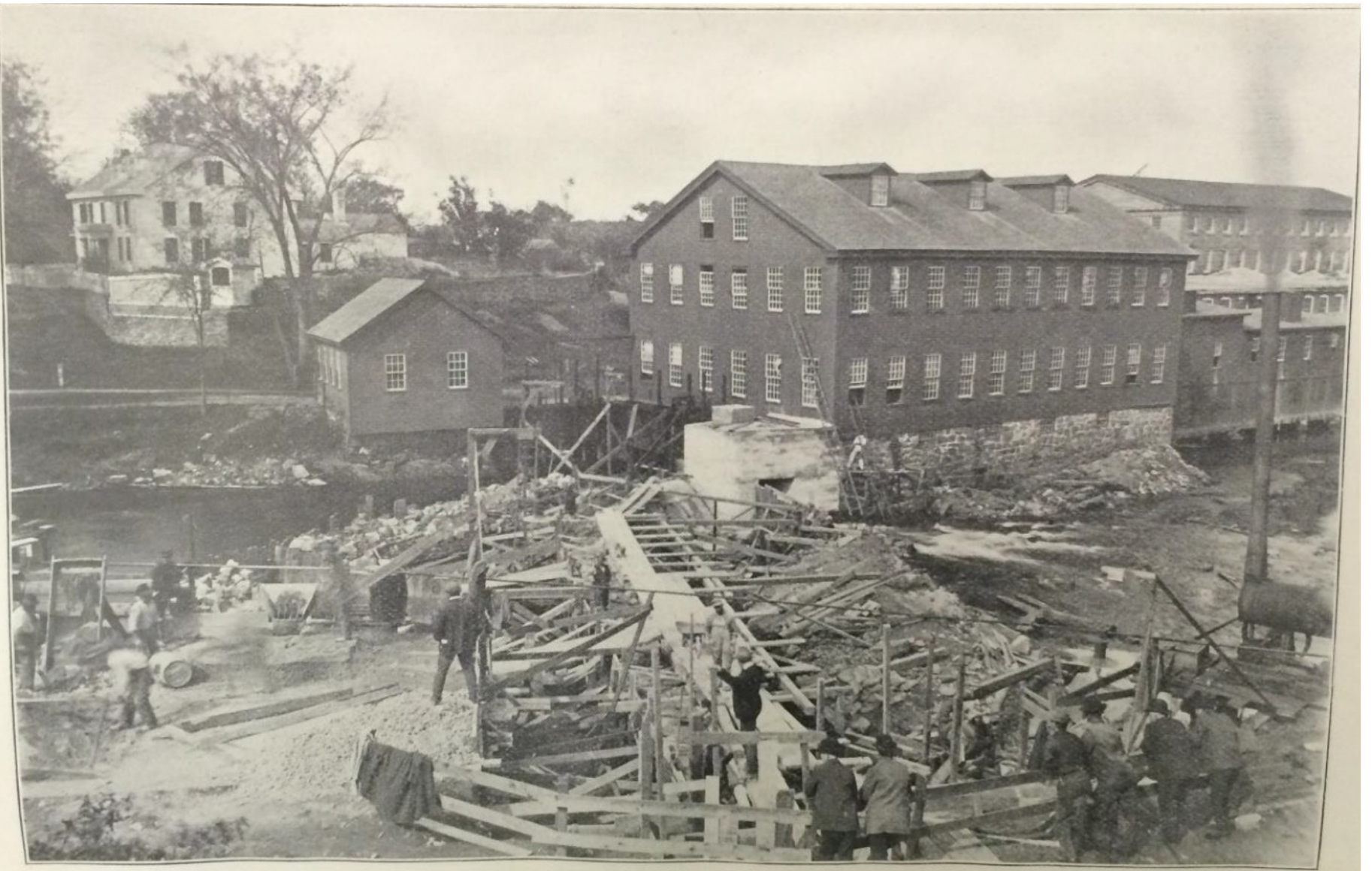
POTTER'S HILL DAM.—Construction of Dam, showing forms and mixer.
